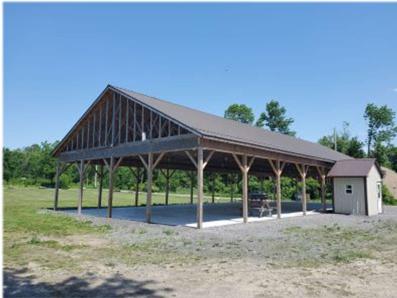
Source: St. Lawrence County Planning Office – Boat Launch Pavilion
