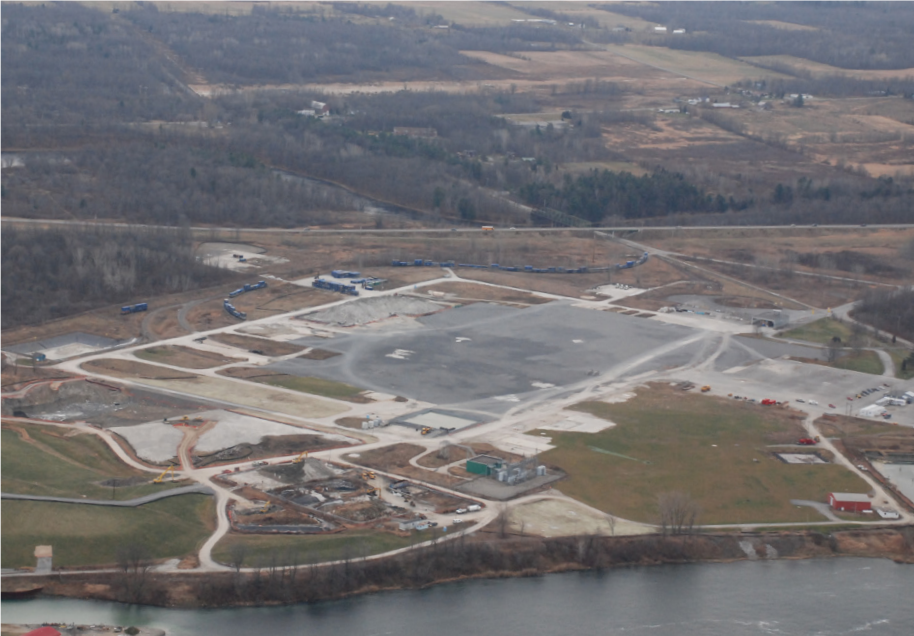
Figure 4. Aerial view of Study Area (2013)
