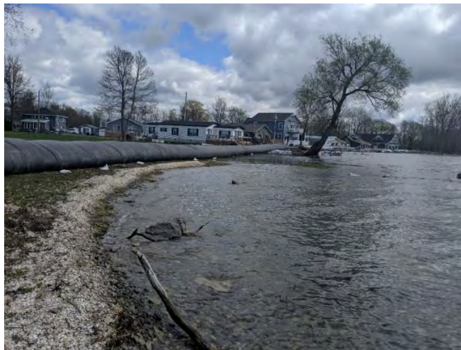
Figure 3.22 – Emergency response measures (e.g., Aquadam and supersack installation) may be warranted to protect properties that are not resilient
