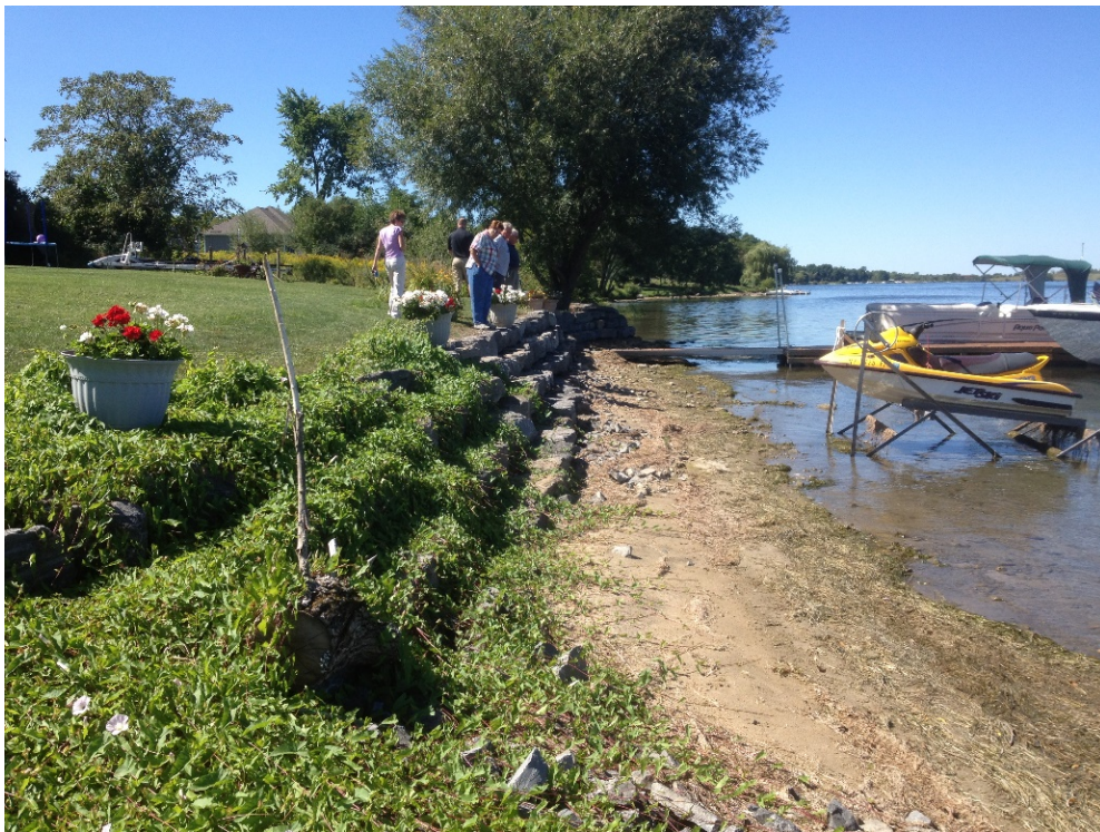
Figure 3.23 – Hard and soft mitigation combined, using limestone blocks and natural vegetation to create a resilient shoreline
