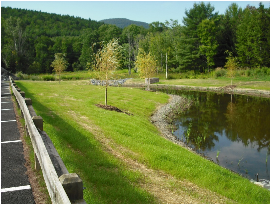
Figure 3.32 – Porous asphalt pavement and low-lying vegetation and retention pond: parking lot system
