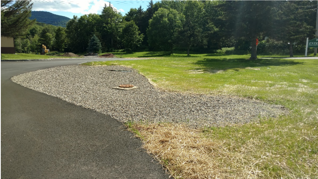
Figure 3.33 – Porous asphalt pavement and recharge bed for water infiltration
