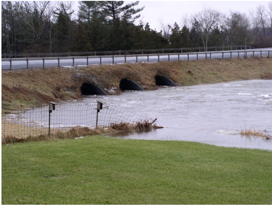
Figure 2.54 – Town of Hammond, Chippewa Bay critical culverts
