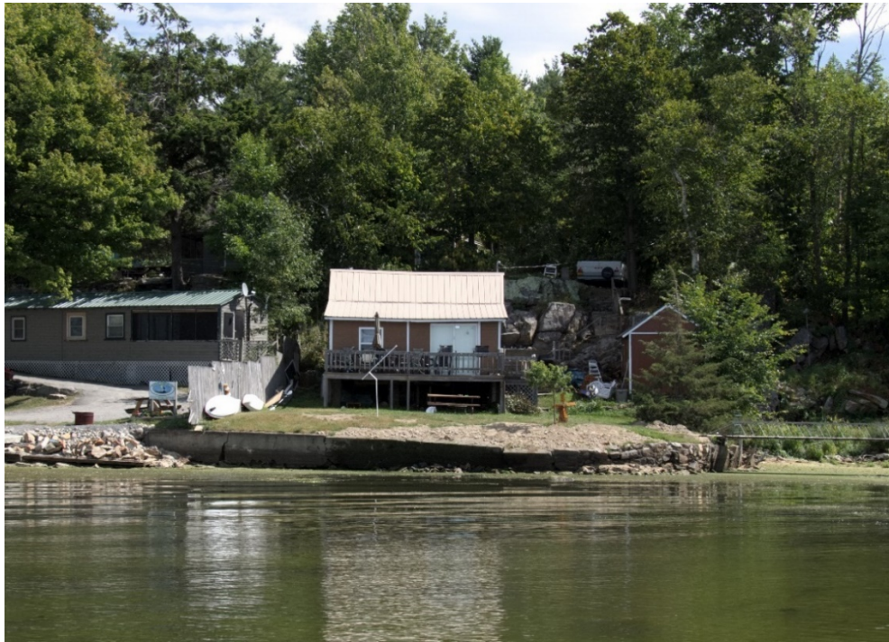
Figure 3.11 – An example of a hardened shoreline which may provide more hazards than benefits in the long term; erosion above the wall may be exacerbated during flooding
