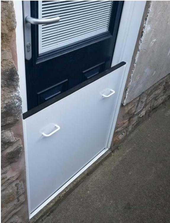
Figure 3.26 – Residential flood gates are used to protect openings (Image courtesy of Stormguard Floodplan)
