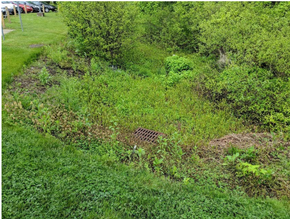
Figure 3.13 – Incorporating more pervious surface systems like this rain garden -or other Green Infrastructure- is a sustainable and Low Impact Development practice
