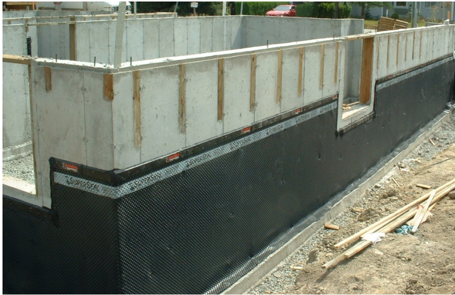
Figure 3.27 – Waterproof membrane used to protect concrete foundation (Image courtesy of SUPERSEAL Construction Projects)
