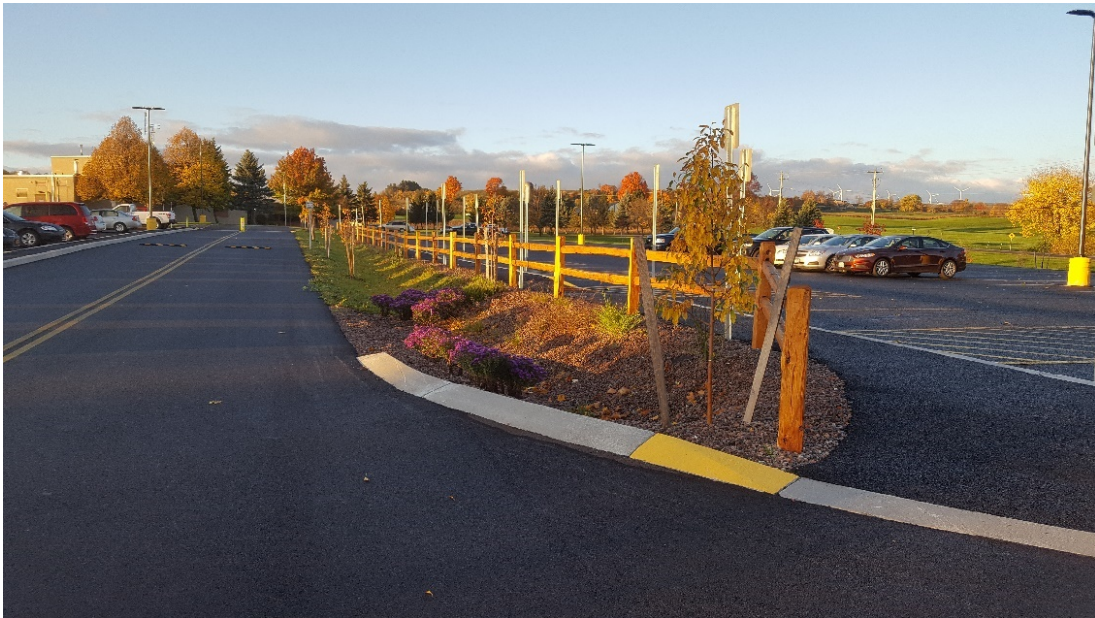
Figure 3.35 – Porous asphalt pavement and bioretention cell to reduce impervious surfaces and make a parking lot area more sustainable
