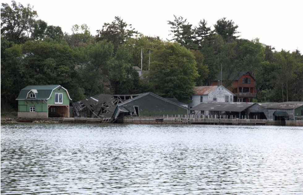
Figure 2.56 – A building constructed directly on the waterfront suffers damage and collapse
