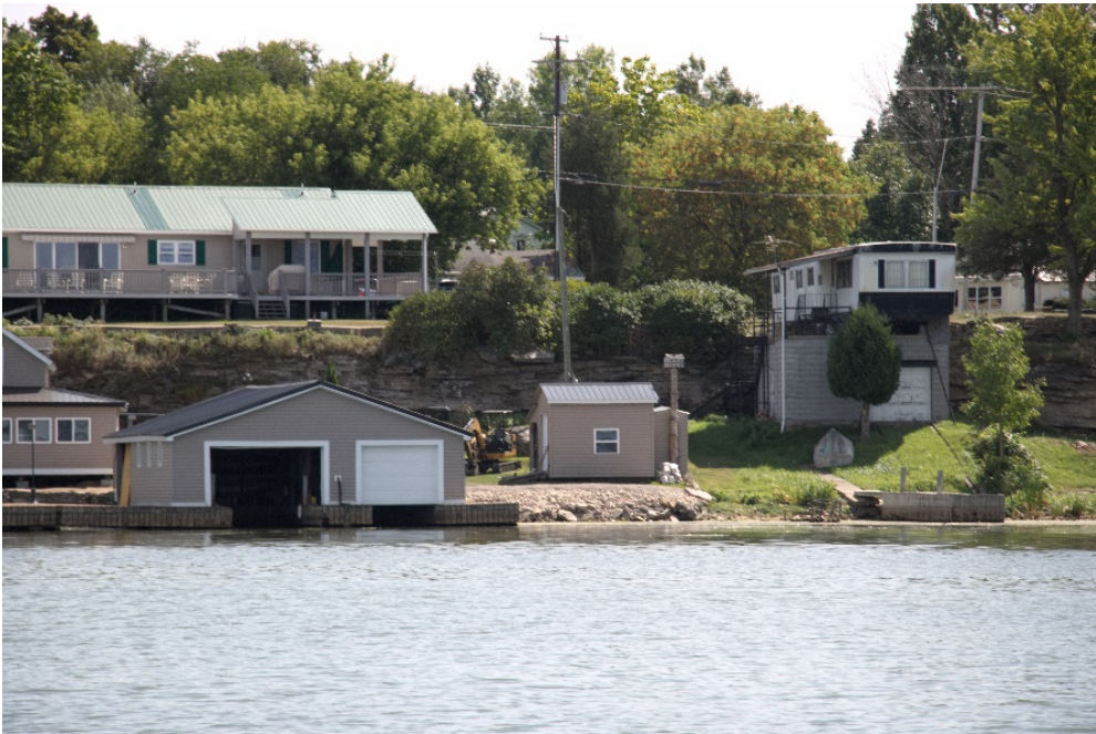
Figure 2.57 – A vulnerable boat garage and shed, juxtaposed with a greatly elevated residential structure
