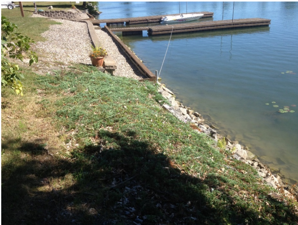
Figure 3.21 – Use of riprap and structural shore walls, as well as natural vegetative features
