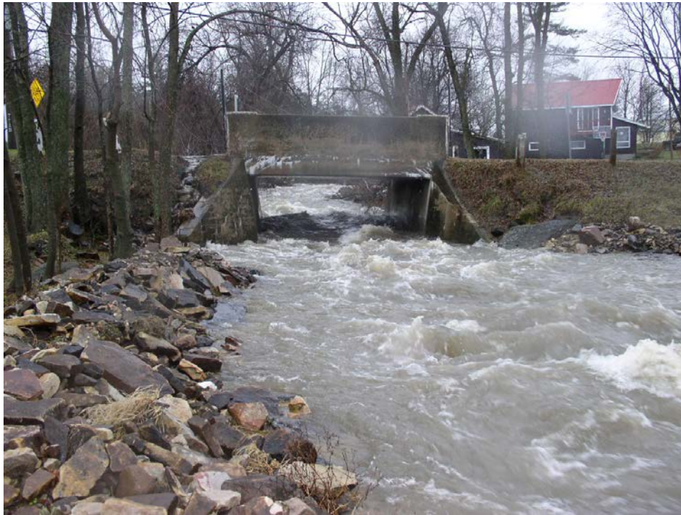
Figure 2.55 – Town of Hammond, Chippewa Bay critical bridge
