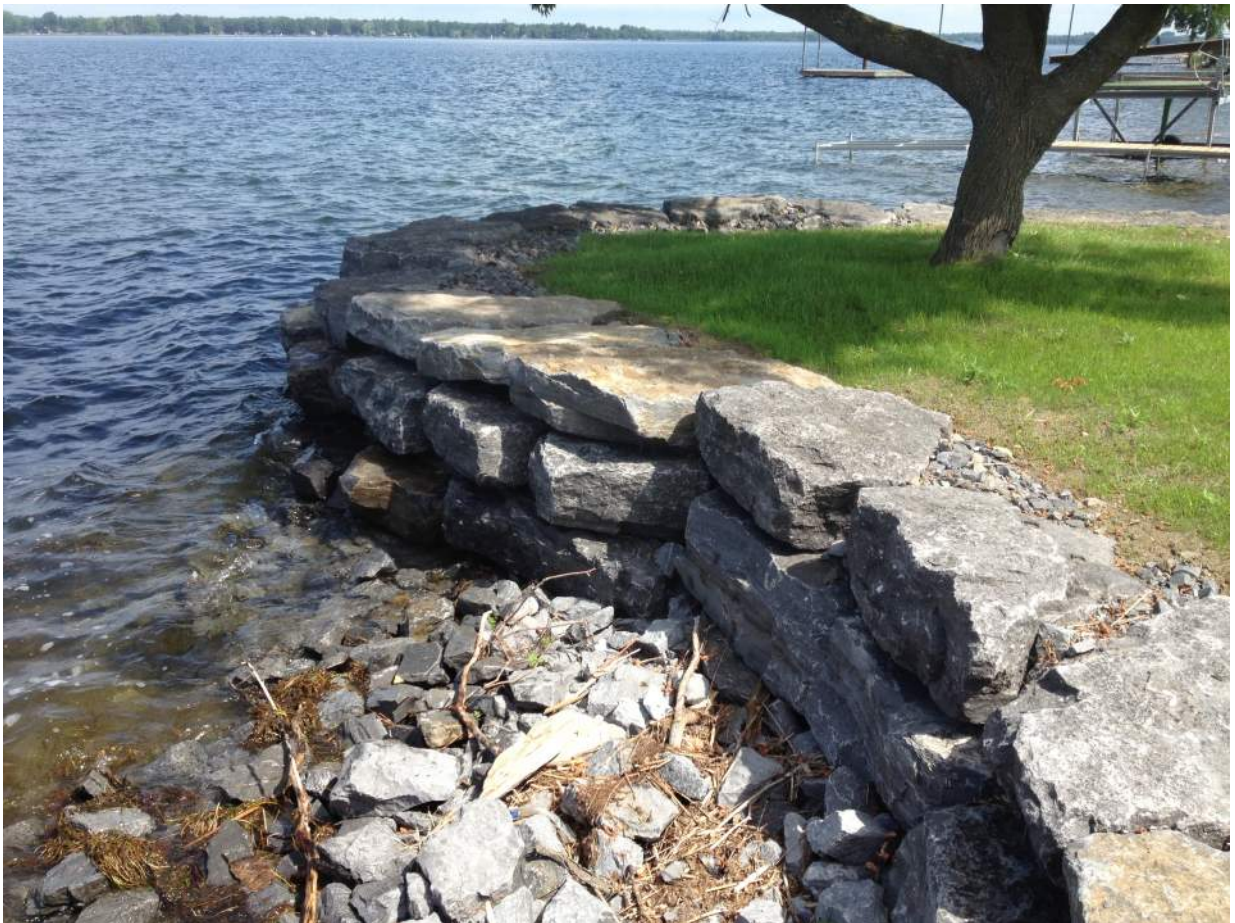
Preserving vegetation is critical to shoreline resiliency - this example shows a stone retaining wall designed around an existing tree to make use of its sturdy root system as part of the shoreline
